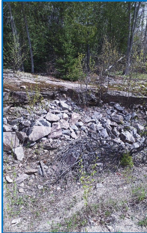
Figure 20: Representative photo of the rock fill placed along the edges of the parking lot.
