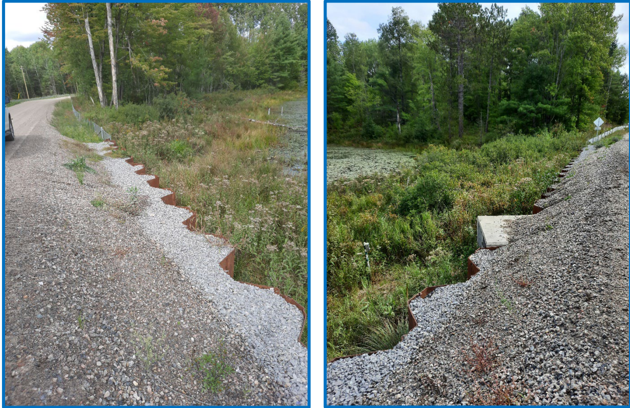
Figure 23 & Figure 24: Example photos of a suitable permanent exclusion system to prevent reptile movement west of the engineered catchment pond.
